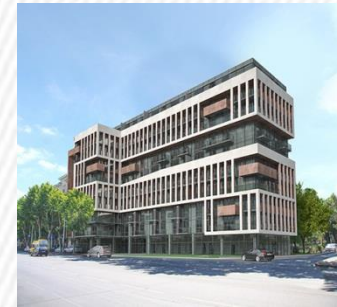
Apartment building: Chavchavadze Avenue Completion status: 1%
