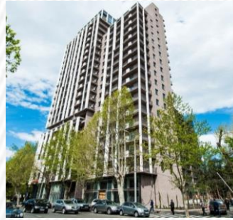
Apartment building: Kazbegi avenue Completion status: 100%
