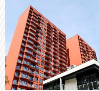
Apartment building: Tamarashvili Street II Completion status: 100%
