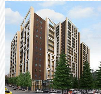
Apartment building: Kazbegi avenue II Completion status: 7%
