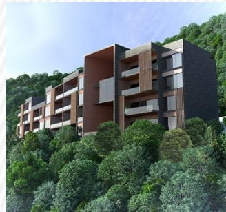
Apartment building: Skyline Completion status: 56%
