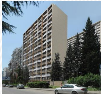
Apartment building: Kartoza Street Completion status: 21%
